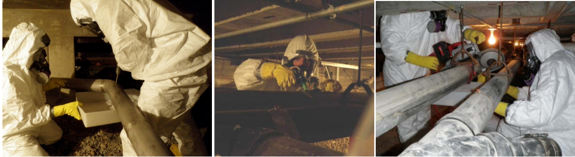
Figure 4: Inserting expanding foam, drilling a hole, and cutting a drain line with a band saw
