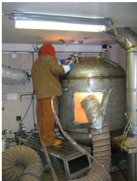
Figure 1: Sectioning UTS tank in-situ tank at the bottom of the tank
