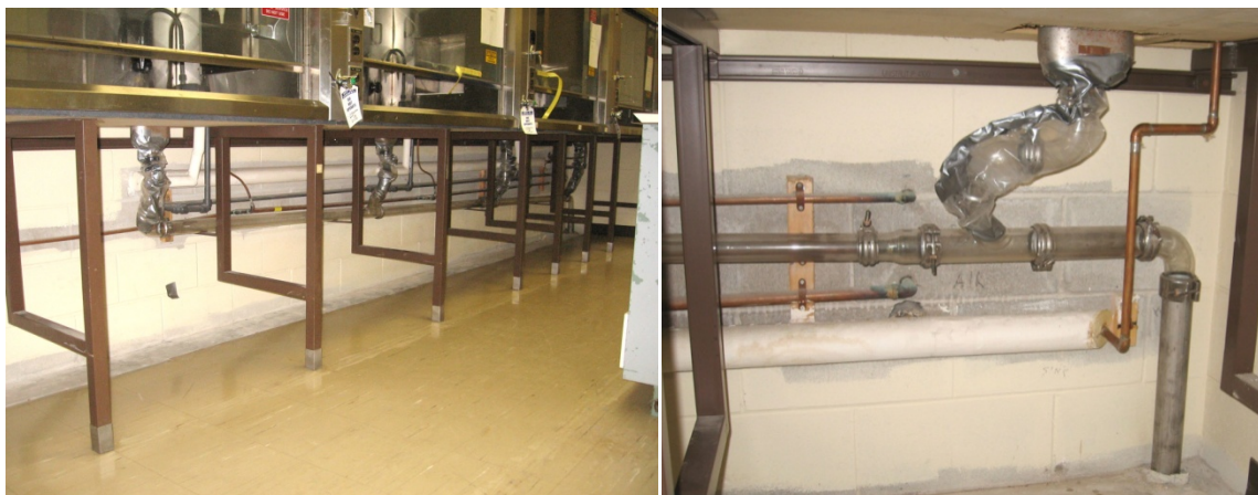
Figure 3 Drain lines under fume hoods and a close-up of a modified glove bag on a glass drain line
