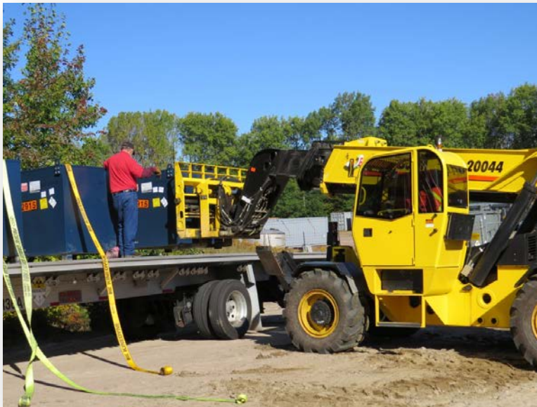
Fig.7 Loading of transport packages for off-site shipment.
