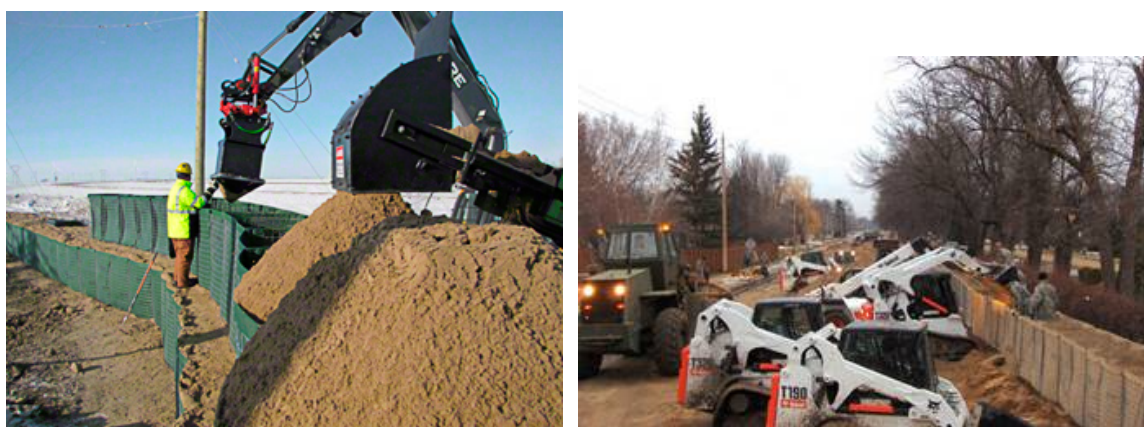
Figure 8. For the HESCO standard container systems a skid loader (bobcat) is used or they have a specialized hopper system with conveyor that directly feeds material into the bags.
