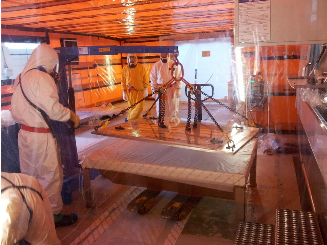
Figure 13 Loading contaminated skip section into milling machine
