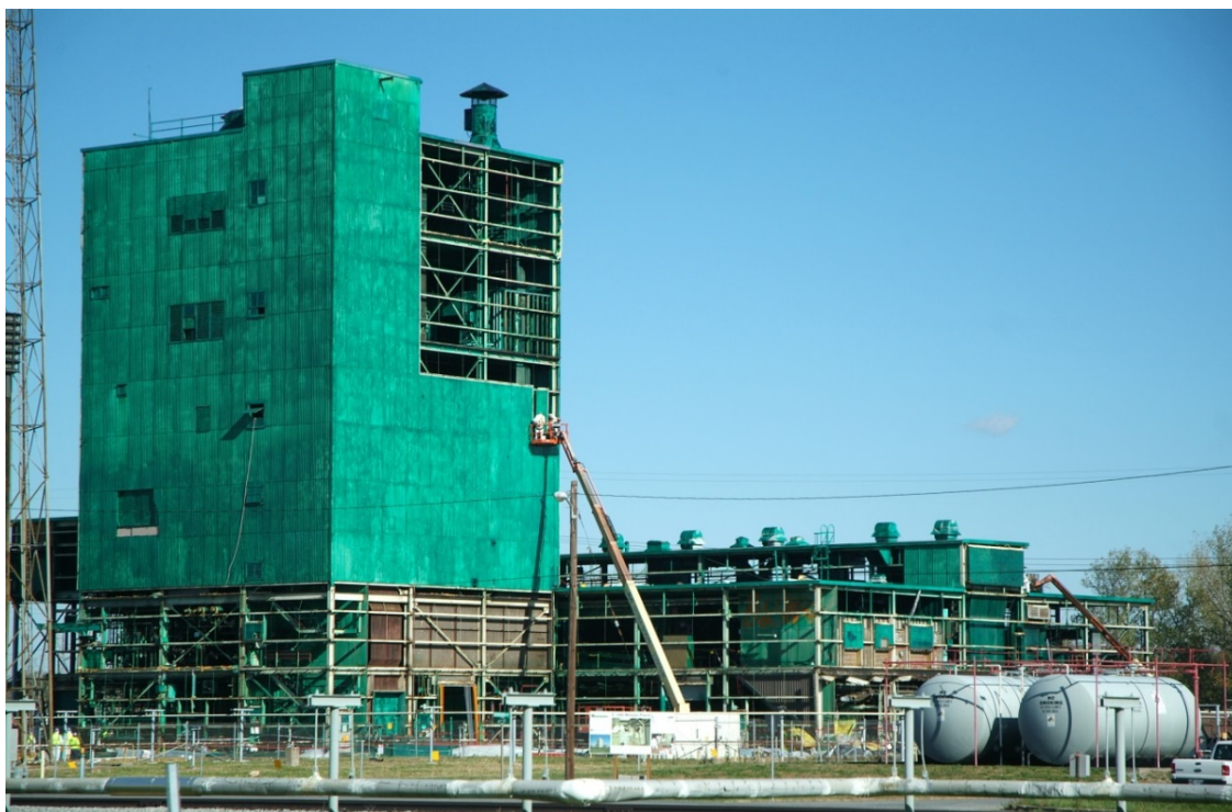
Figure 2. Transite Removal at the C-340 Metals Complex
