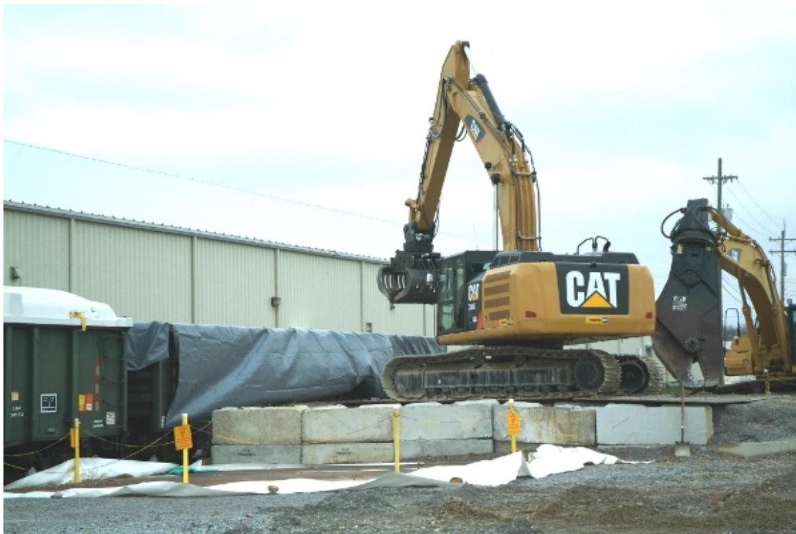
Figure 3. Downsizing (background) and Loading C-340 Debris into Gondolas
