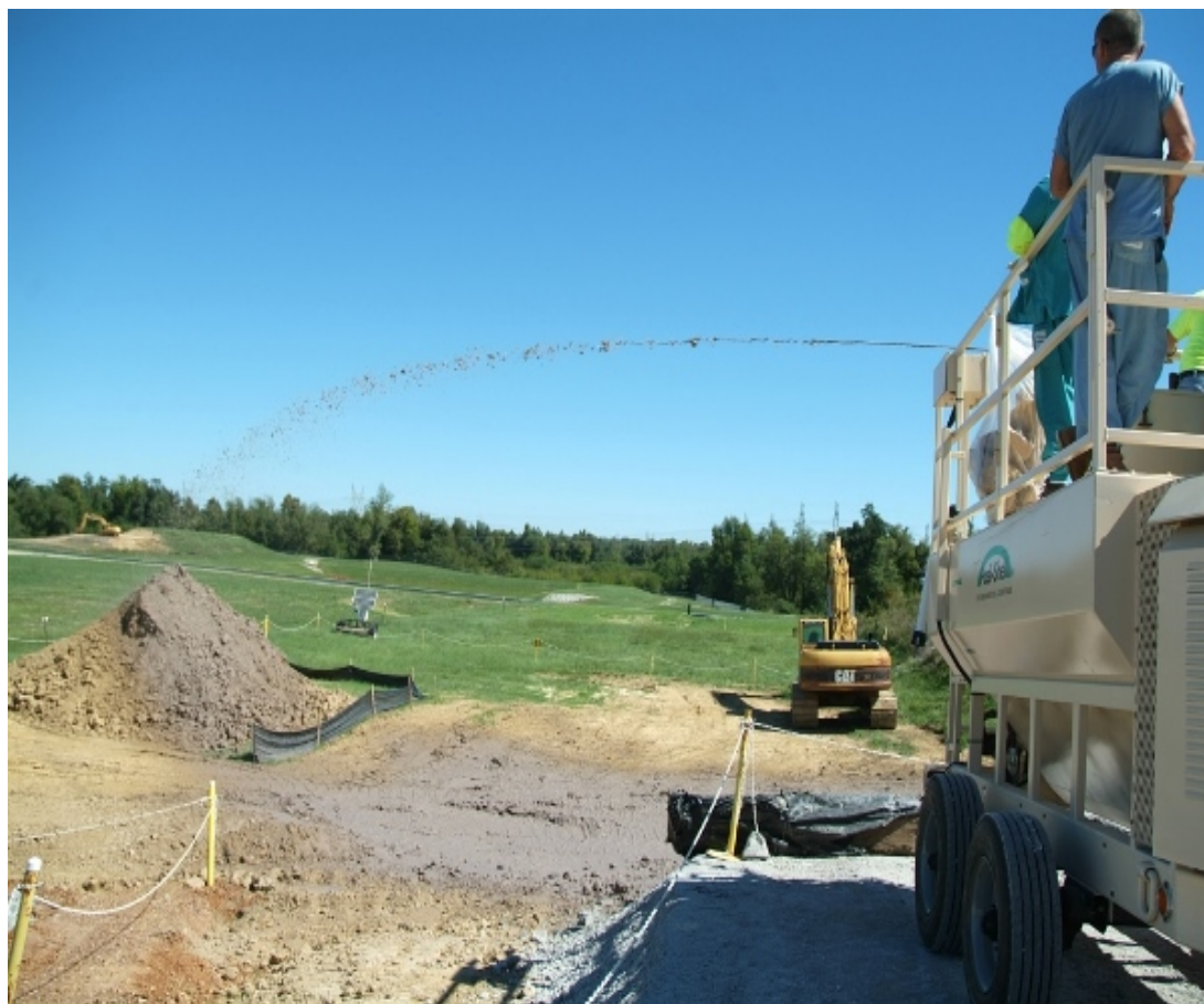
Figure 4. Workers Being Trained to Apply Posi-Shell Alternative Waste Cover Using a Hydroseeder
