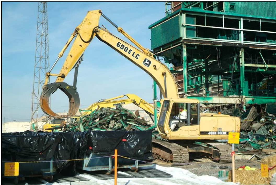
Figure 2. Waste is Loaded Directly into Shipping Containers in Areas Adjacent to C-340
