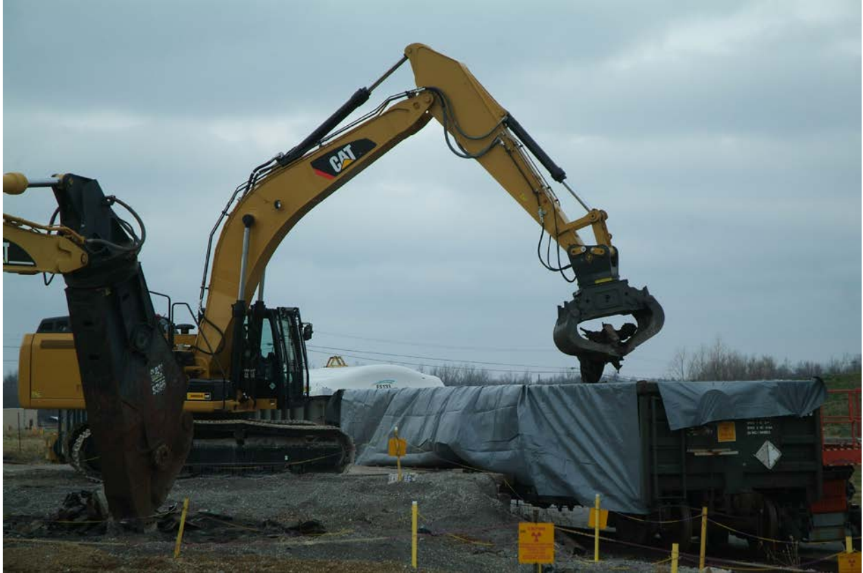
Figure 5. Heavy equipment was used to cut large steel sections into smaller pieces so that rail cars could accommodate more waste
