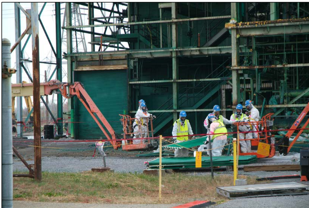
Figure 3. Staging of Transite after Removal from the C-340 Complex
