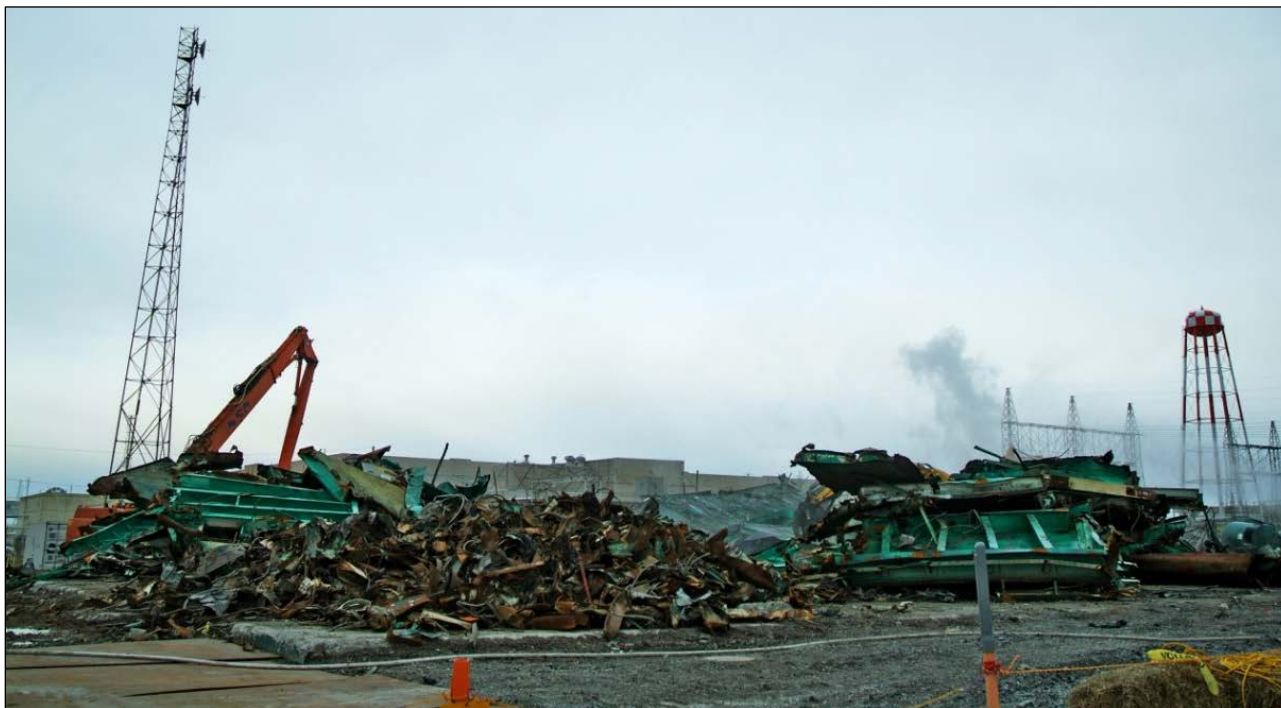
Figure 4. Debris Is Being Sorted into Waste, Part of Which Will Be Shipped to an Approved Disposal Facility and the Rest Taken to the On-site C-746-U Landfill
