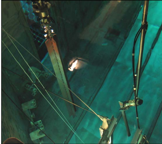
Fig.13. Cutting of control rod shafts.
