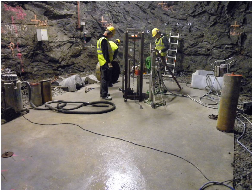
Fig. 4. Drilling of the first demonstration hole.
