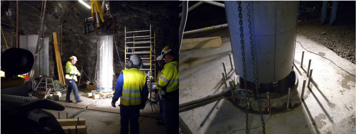
Fig. 10. Block stacks above the holes and the beginning of block stack installation.
