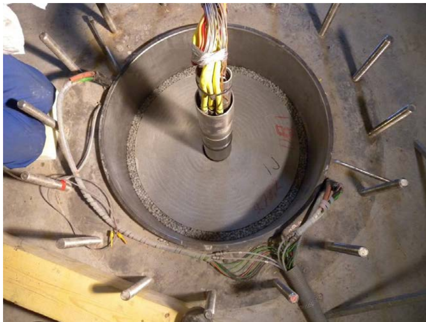
Fig. 11. The installed pellets in the hole 2.
