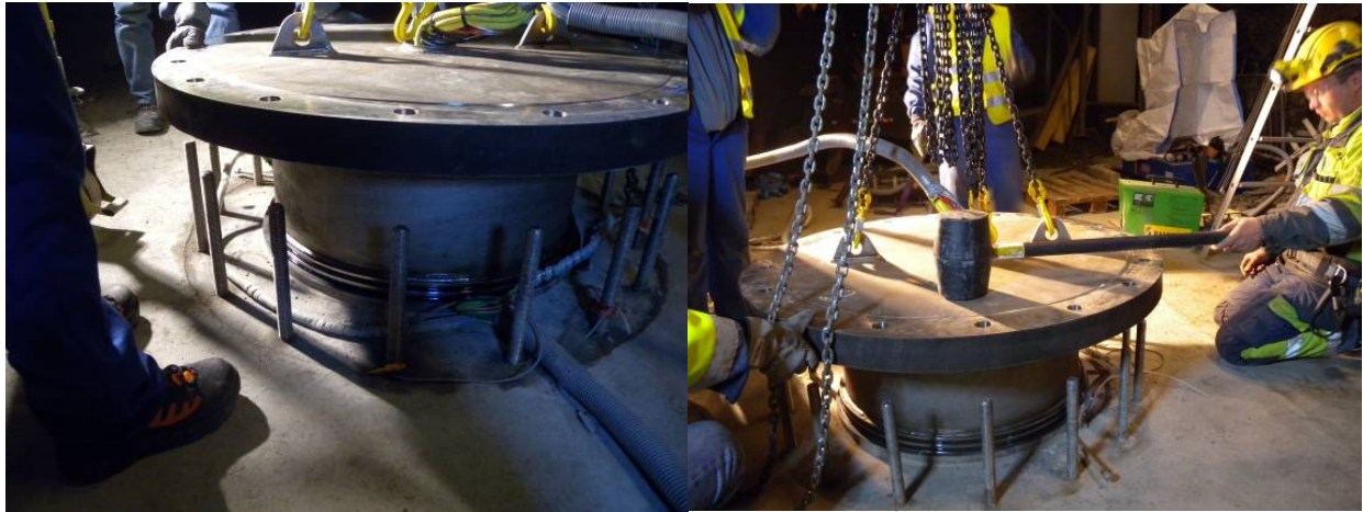
Fig. 12. Installation of piston and adjusting by rubber sledgehammer.
