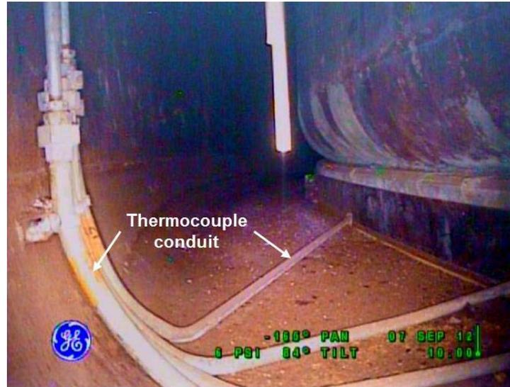
Fig. 4. Thermocouple conduit pipe located on the annulus floor between Riser 91 and Riser 83.
