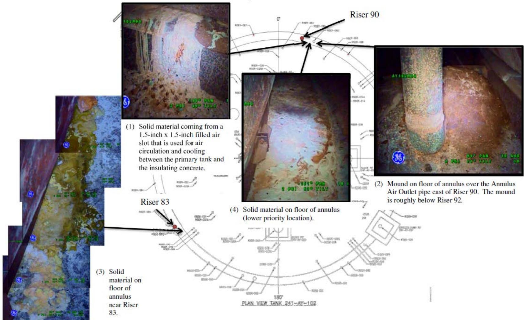
Fig. 1. Images taken of the unknown solids with arrows pointing to their general locations in the annulus on a plan view diagram of tank 241-AY-102.
