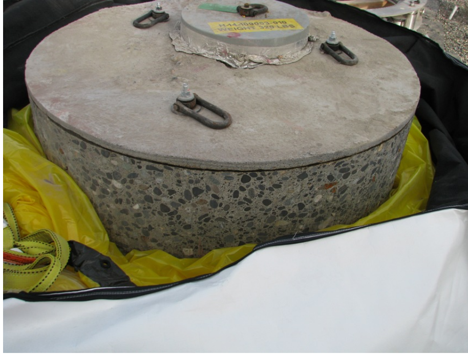
Figure 8. SST 241-C-107 Dome Plug
