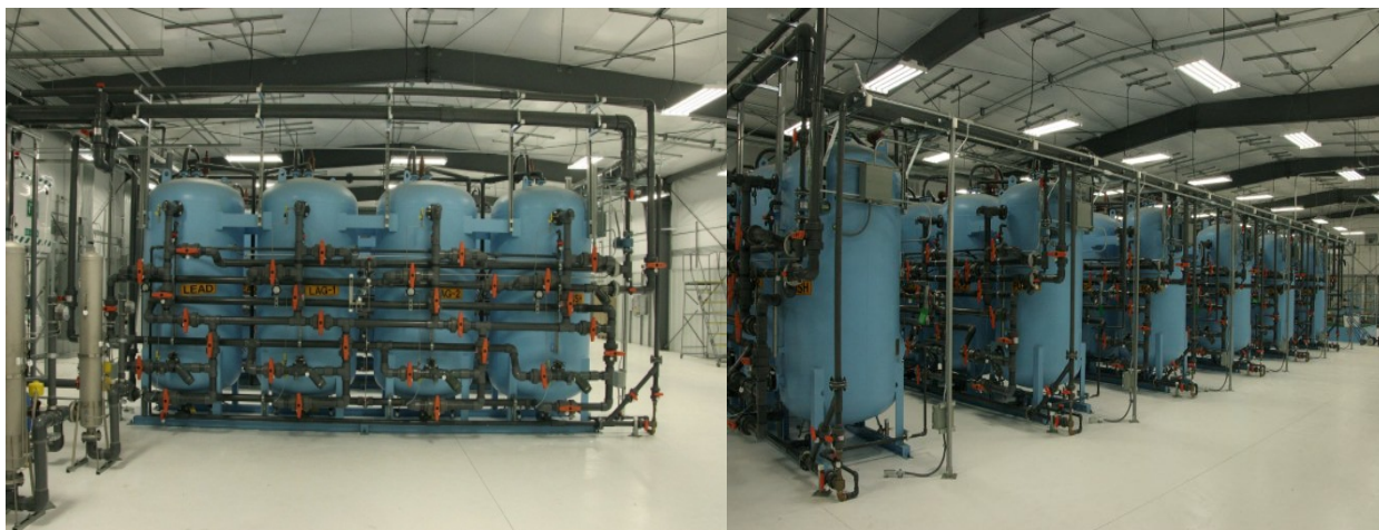
Fig. 3. Ion Exchange trains at DX pump-and-treat
