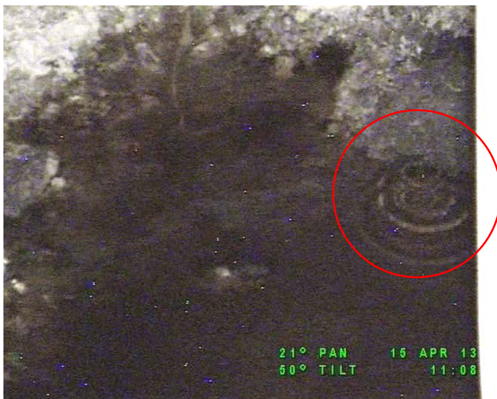
Fig. 4. Tank SX-106 liquid pool ripples.
