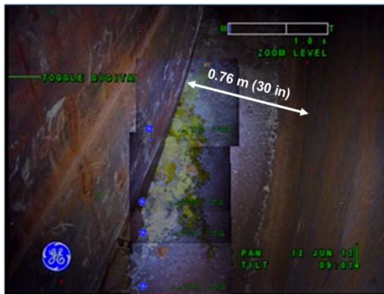
Fig. 5. Tank AY-102 Waste Material Discovered Near Annulus Riser 83
