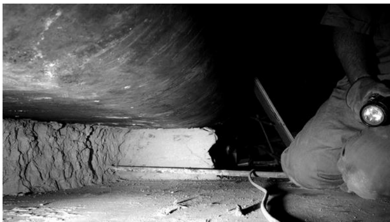
Fig. 7. Tank AY-102 Insulating Refractory Repair: Preparation for Placement of Reinforced Concrete
