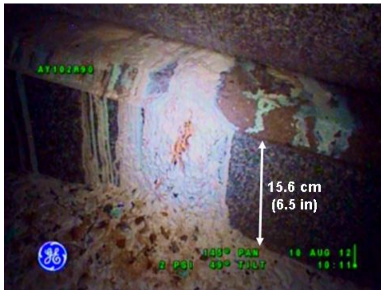
Fig. 4. Tank AY-102 Waste Material Discovered Near Annulus Riser 90
