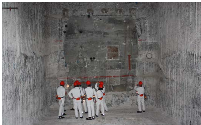
Fig. 1 Drift seal in the low and intermediate level radioactive waste repository Morsleben – 484 m 3 salt concrete M2 in a construction of 4 – 5 m height, 4.5 m width and 25 m length
