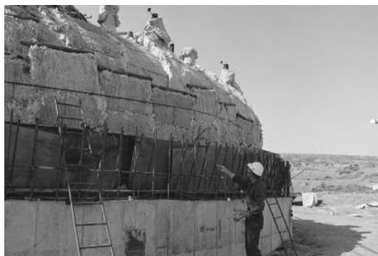
Insulation Prior to Heat Treatment
