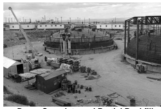
Dome Complete and Partial Backfill
