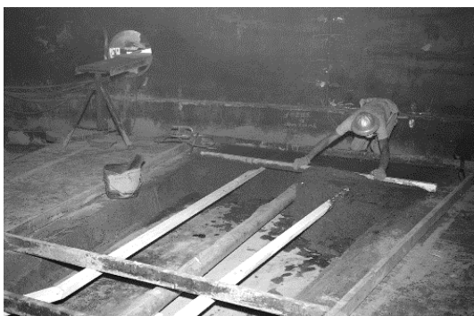
Installation of Refractory
