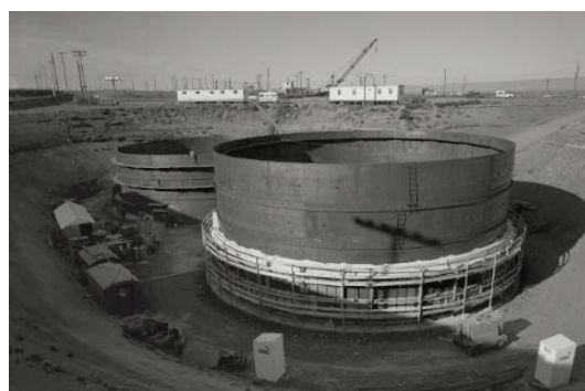
Erection of Secondary Liner and Concrete Wall
