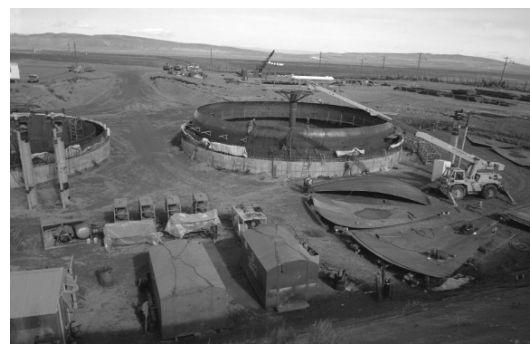
Erection of Dome Plates
