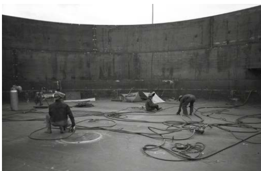
Fabrication of Primary Bottom
