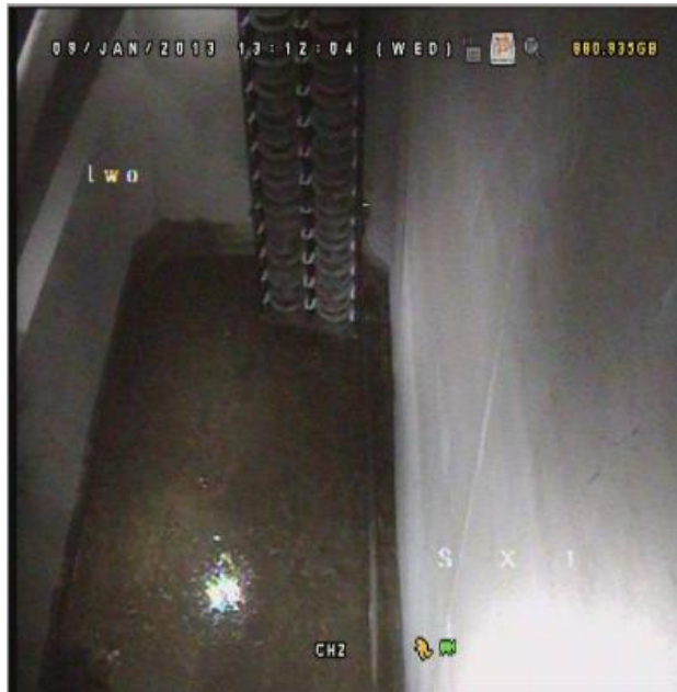
Fig 4. Buffer store installed in PNV.
