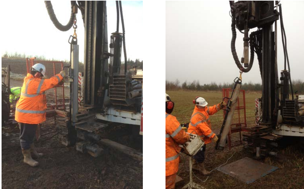
Figure 8 - Use of casing handling tool
