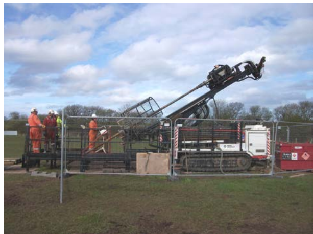
Figure 6 - Vertical and inclined boreholes being drilled using coreless 'lost cone' technique
