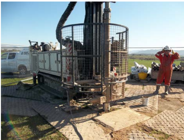
Figure 6 - Vertical and inclined boreholes being drilled using coreless 'lost cone' technique
