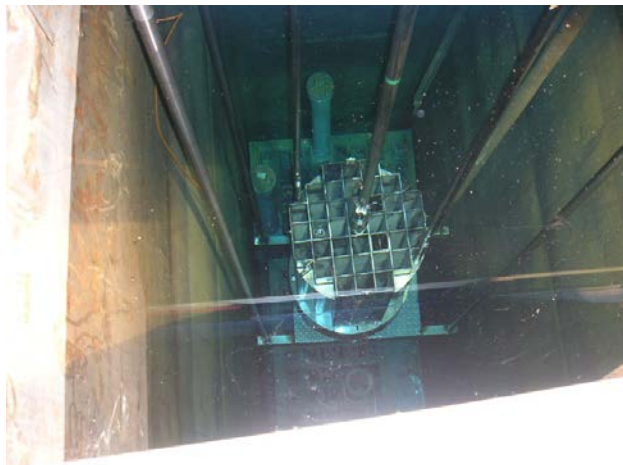
Fig. 4. Loading SNF inside the pool into the basket
