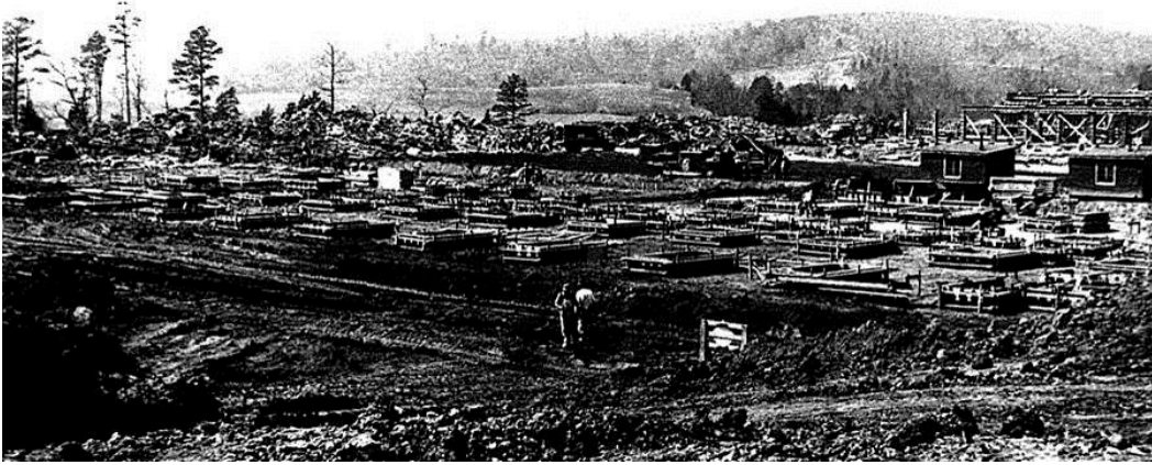
Fig. 1. K-25 footings, April 6, 1944.
