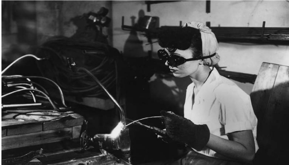
Fig. 5. Worker performing air tight welding.
