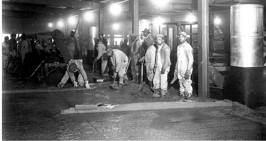
Fig. 3. Workers pouring monolith floor slab on operating floor, Feb. 5, 1945.
