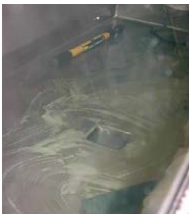
Fig. 6 Cleaning Hot Spots with Rad Release Agent
