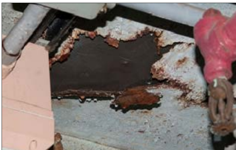
Figure 4. Y-12's Building 9206 Ceiling Degradation
