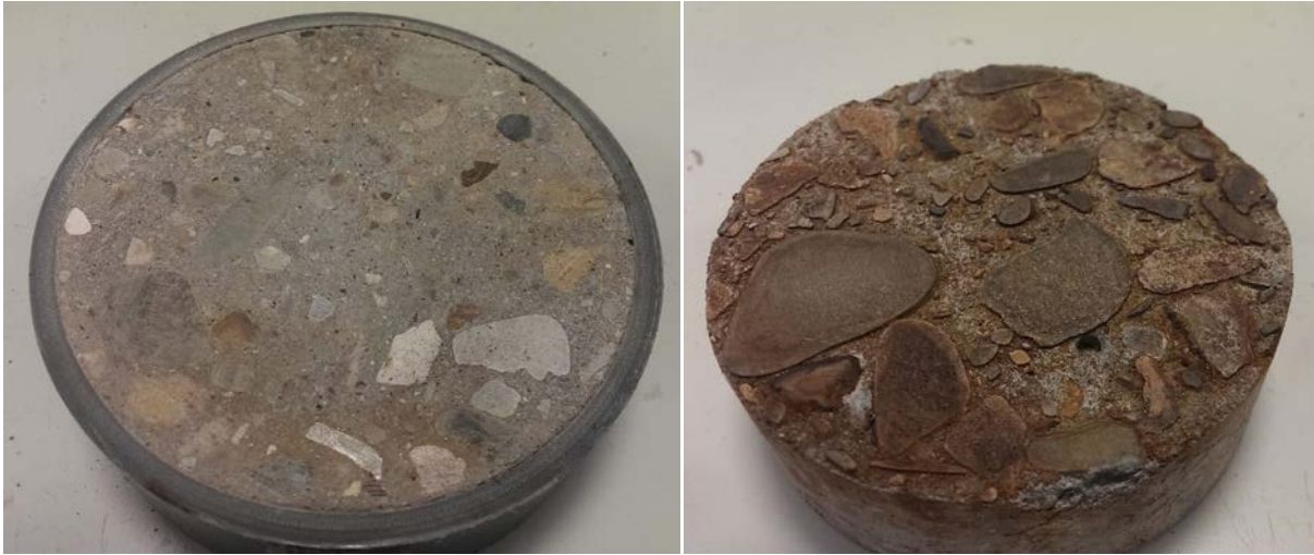
Figure 9. Photographs showing the physical affects that pH control has on the concrete surface, left pH controlled, right uncontrolled.
