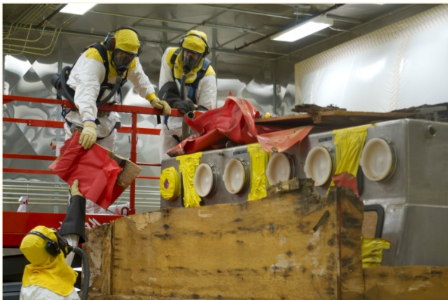
Fig. 3. Remediation of FRP Box in Dome 375 Boxline
