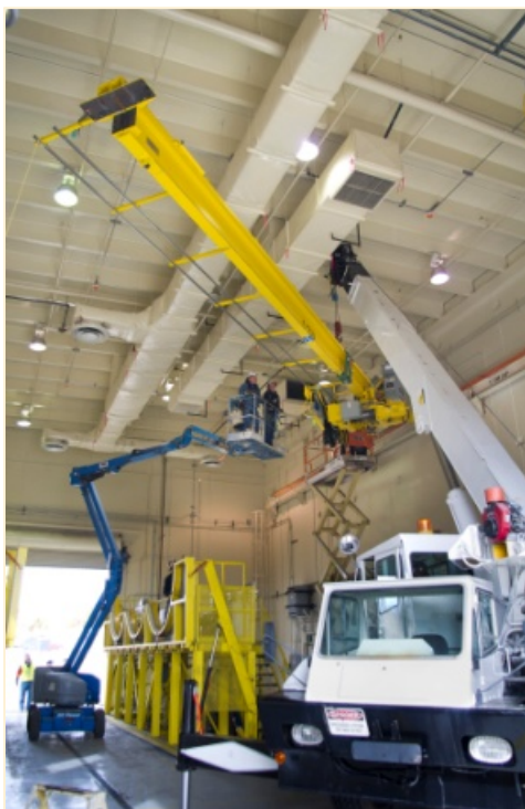
Fig. 4. Installation of Second Crane for TRUPACT-II Loading
