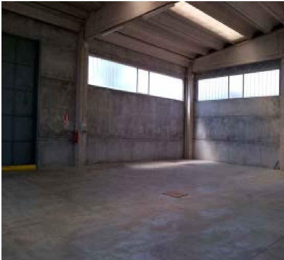
Figure 6 – Controlsonic deposit after the decommissioning.
