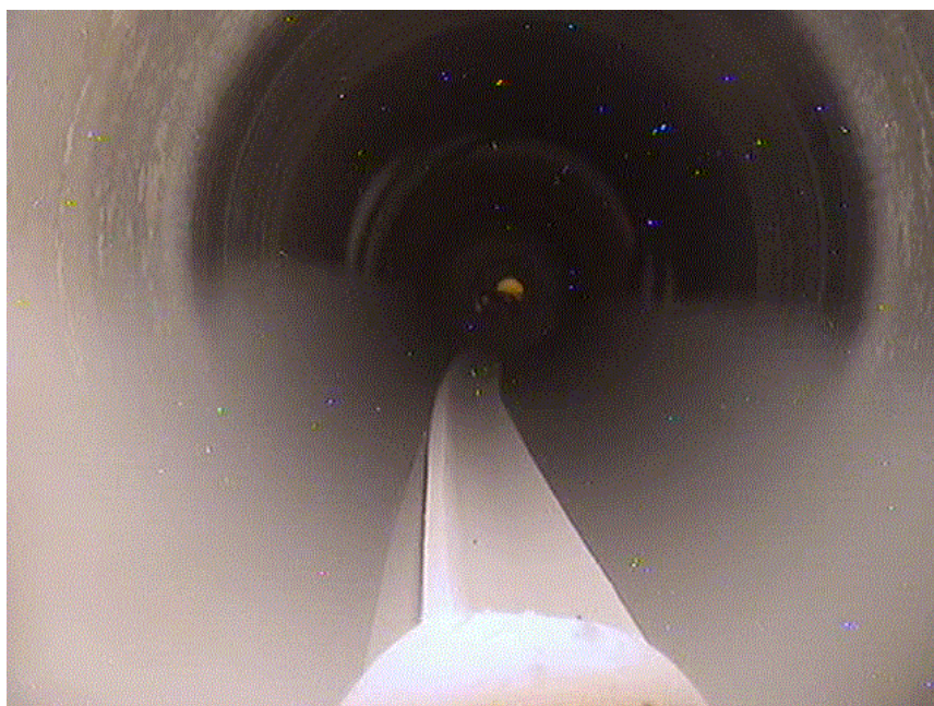
Fig. 5. Interior of the calciner after the campaign
