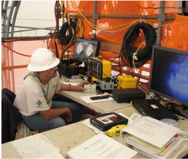
Fig. 1. The dive control station was located on top of steam generators near the entry point.
