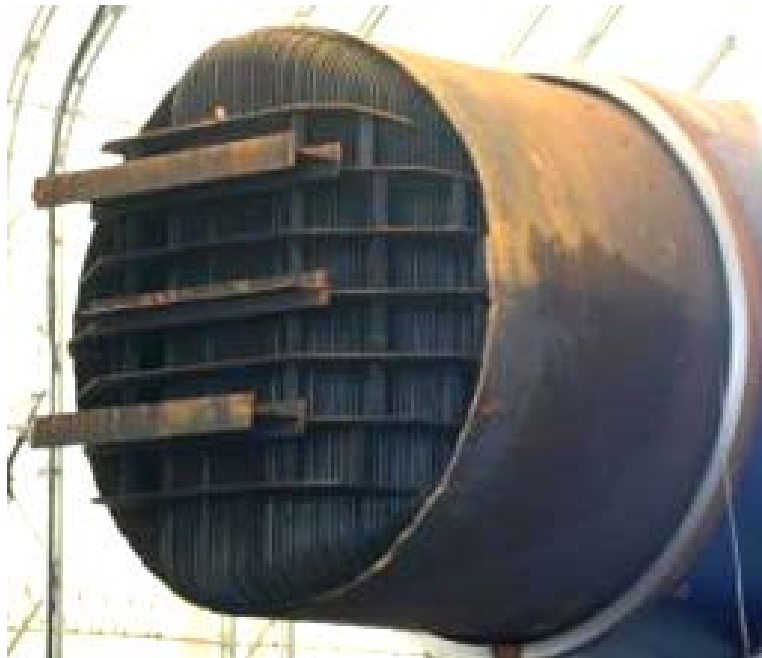
Fig. 14. Severed tube bundle support beams remained attached to the tube bundle on the lower assembly.
