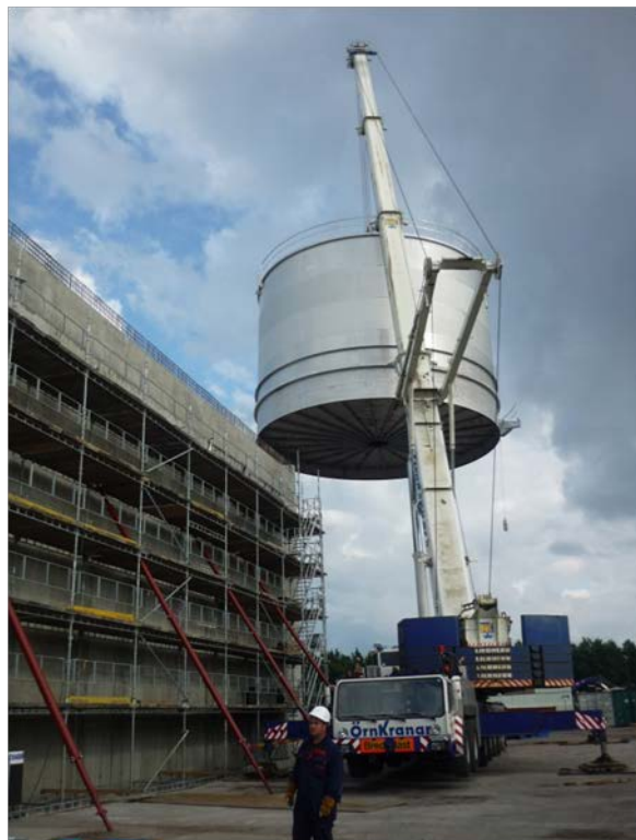
Figure 1: Installation of one of the new 1,500 m 3 buffer tanks at the Forsmark site.
