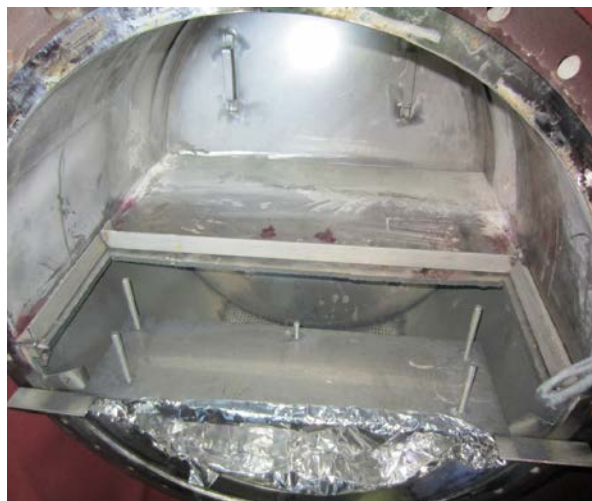
Fig. 5. Section of pass partition plate removed – leaving a 3/4-in piece along the
