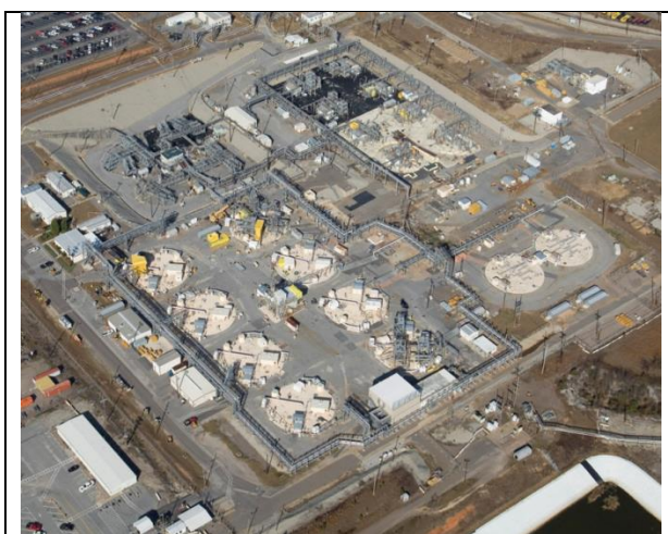
Fig. 2. SRS F-Tank Farm.
