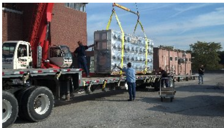
Figure 3: Loading the First Glovebox for On-site Transport
