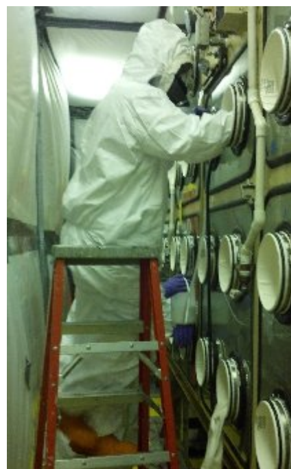
Figure 1: Workers spraying fixative in the glovebox
