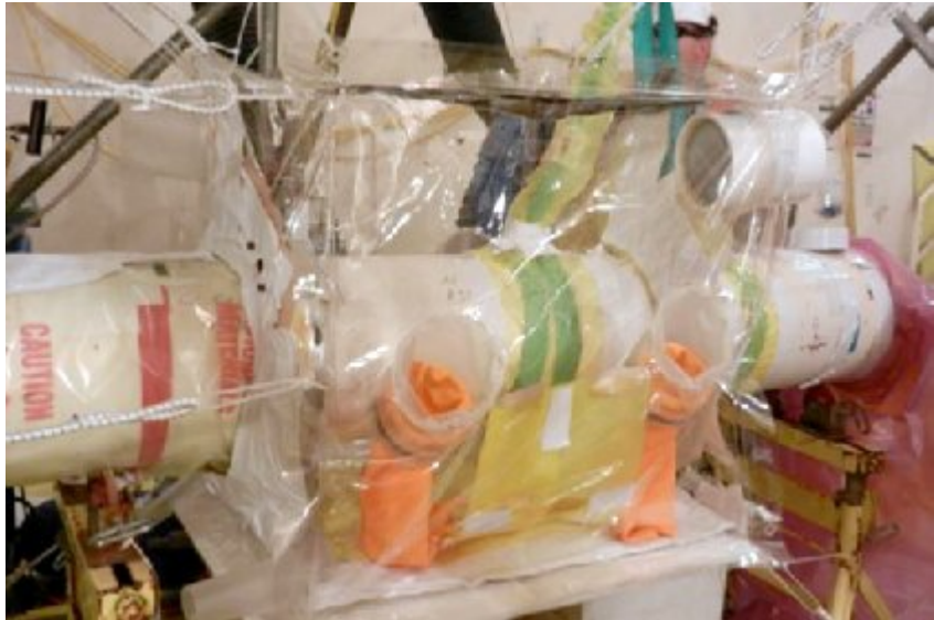
Delicate glove bag operations cutting steam piping
