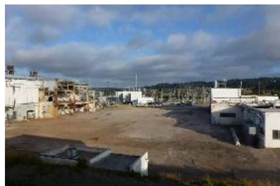
Above grade demolition completed
