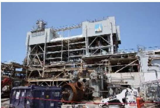
Fossil Units 1 and 2 being demolished
