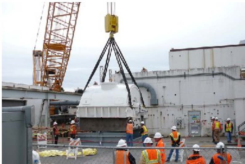
Removal of the Low Pressure Turbine
