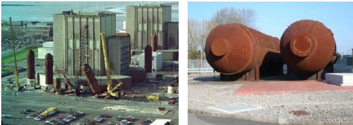
Fig. 2 Photographs showing boiler lowering and final example of one storage location
