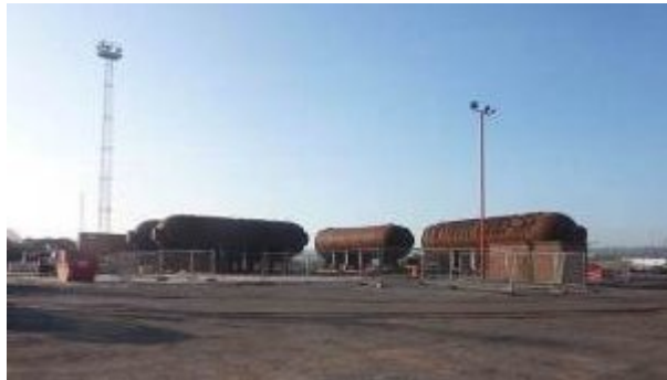
Fig. 7 In-transit storage of boilers
