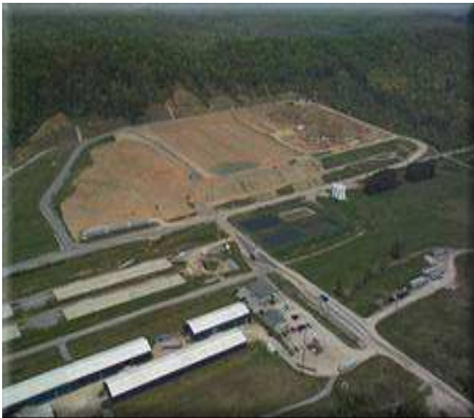
Figure 2. The EMWMF, an onsite disposal facility, has reduced cost and minimized transportation risks.
