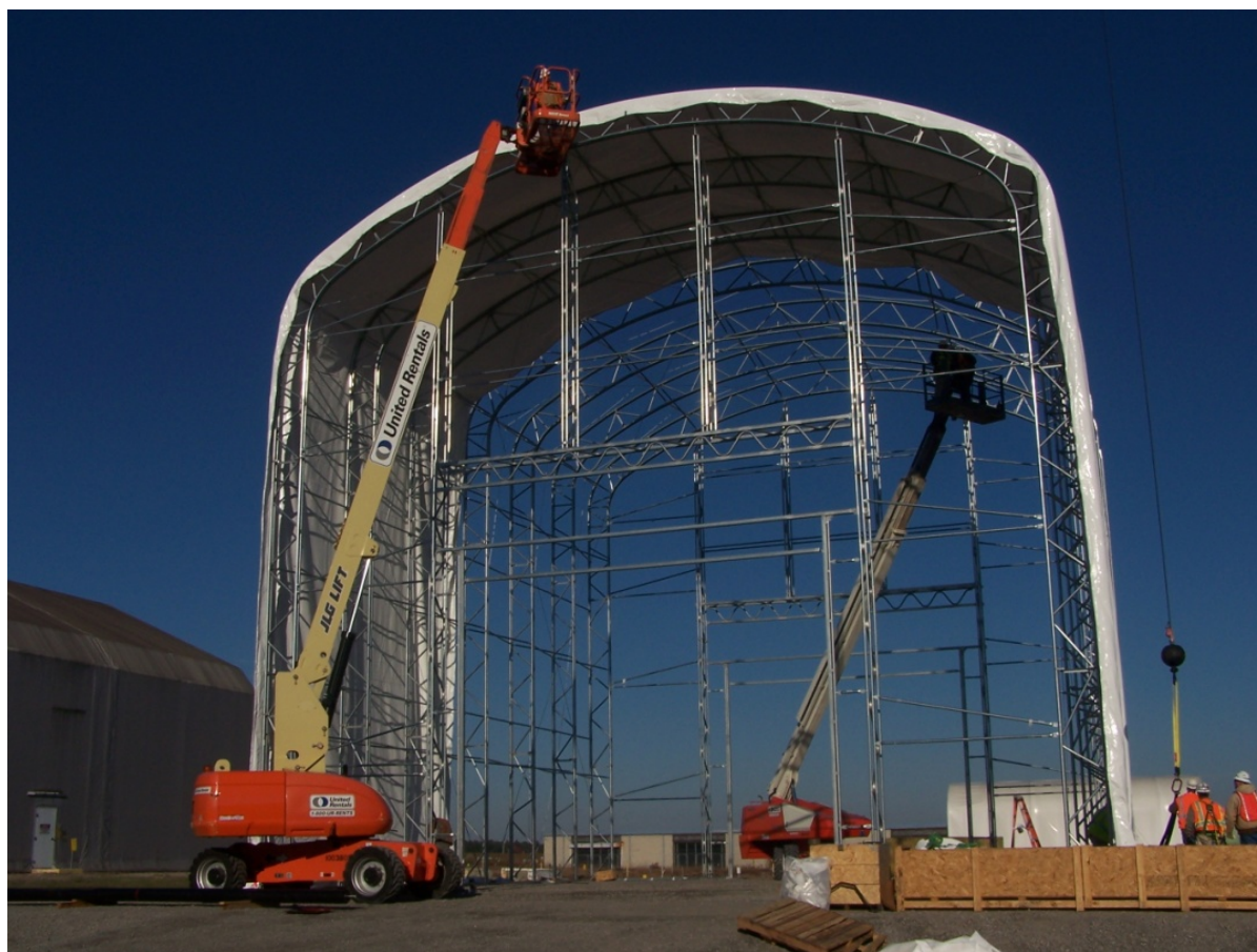
Figure 3 – Construction of 9E Culvert Unloading Facility
