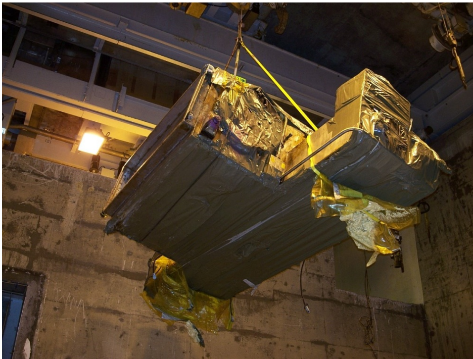
Figure 1 – Legacy Glovebox Being Lifted in H Canyon Truckwell
