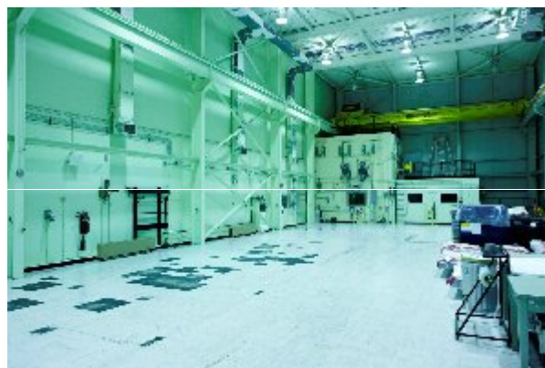
Fig. 3. Area where IFTF Warm Cells were located after decommissioning was completed
