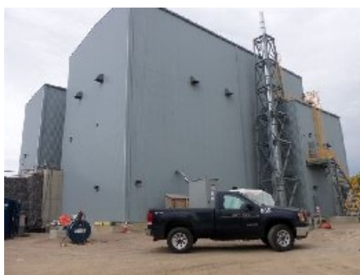
Fig. 1. Fuel drying, repackaging and storage facility at CRL
