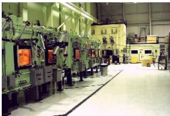
Fig. 2. IFTF Warm Cells before decommissioning
