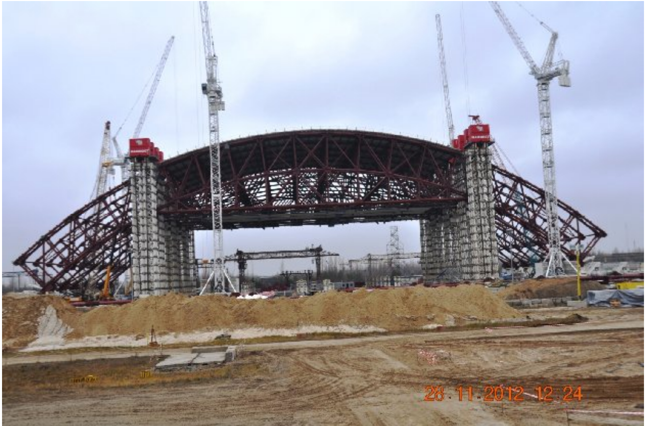
Figure 3 Arch Sections Assembly and the first lift, November 2012
