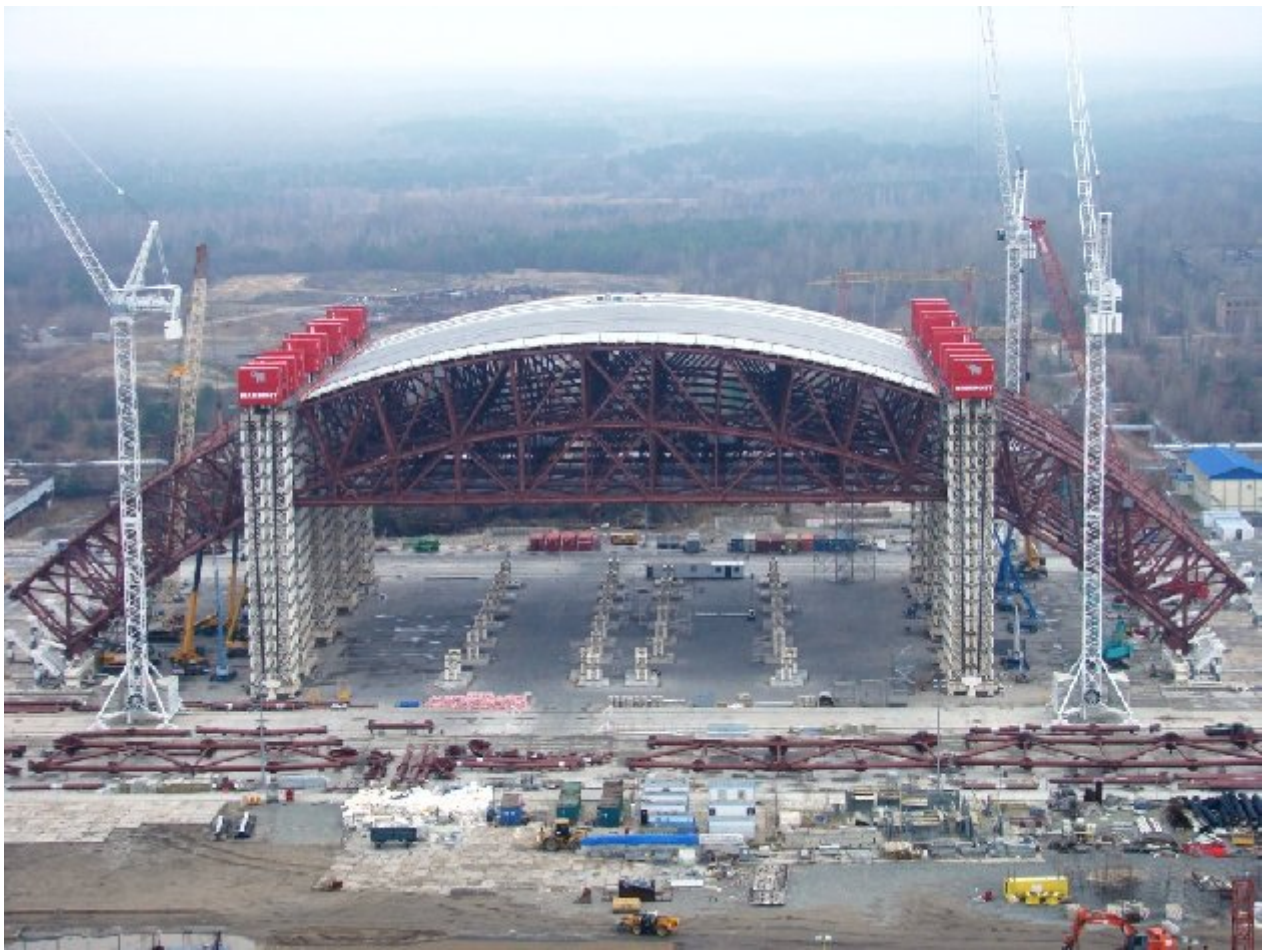
Figure 2 Arch Sections Assembly and the first lift, November 2012
