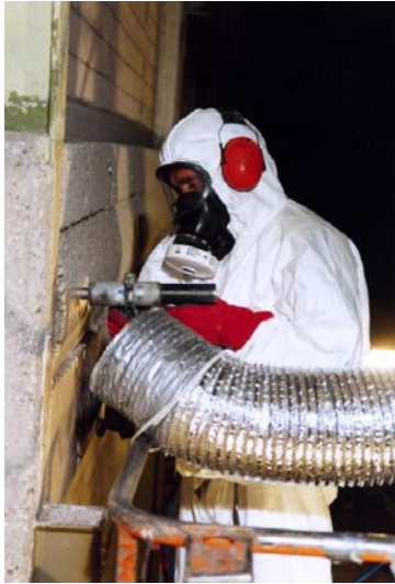
Figure 4: abrasive grit blasting
