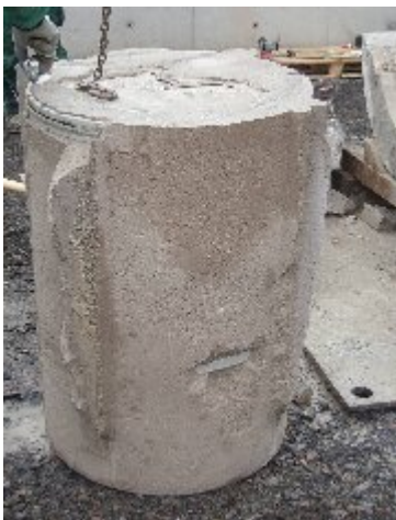
Figure 12: freed drum with concrete
