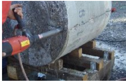
Figure 6: use of the hydraulic splitter
