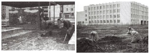
Mechanical decontamination led to the formation of huge amounts of waste. Mechanically econtaminating one hectare generated from 1000 to 1500 tons of radioactive waste. Such amounts needed to be buried, which led to the formation, in areas adjacent to Pripyat and Chernobyl, about 800 "graves", excavated trenches in which were buried radioactive waste.
