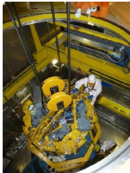
Fig. 15. Preassembling HWZ in the caisson
