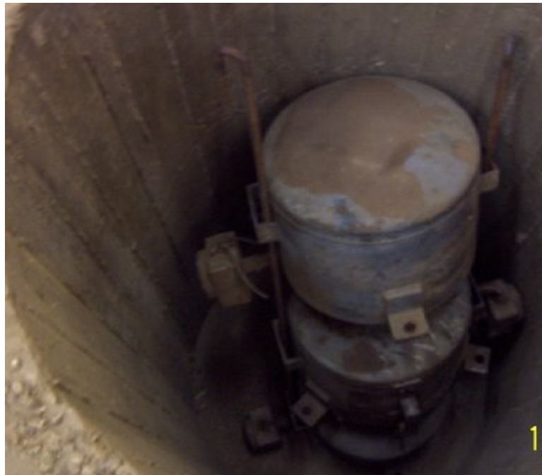
Concrete bunkers for medium and long term storage
