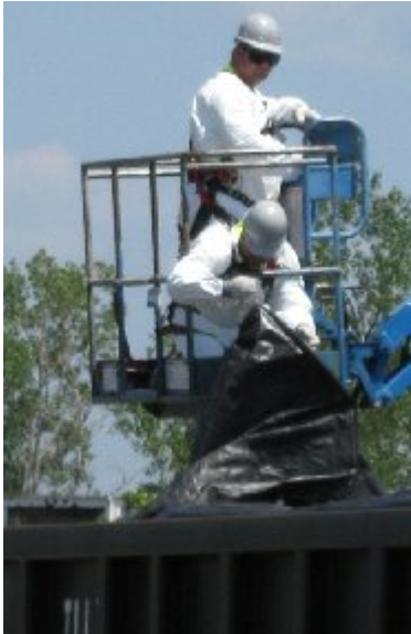
Figures 9 - 10: Liner closure from aerial lift (left). Lift chasis outside of the loading area (right).
