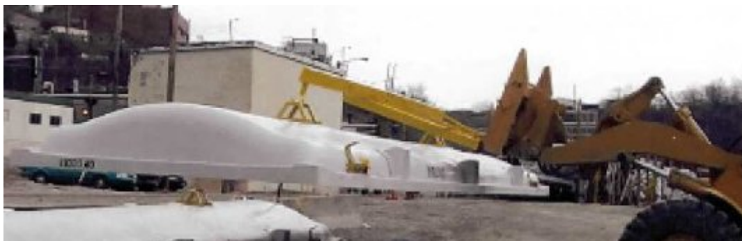
Figure 13: Hard cover suspended from loader and lifting frame.
