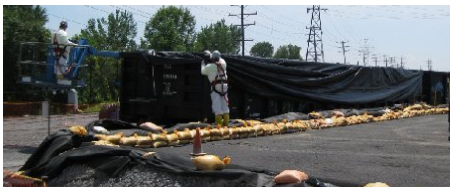
Figures 1 - 2: Lined railcar interior (left). Liner installation assisted by aerial lift (right).
