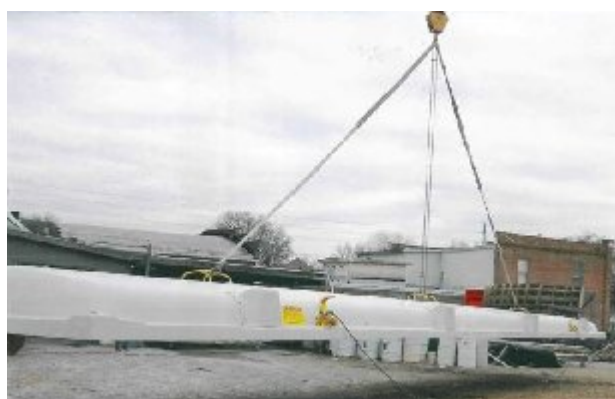
Figure 14 - 15: Placement with all-terrain forklift (left). Hard cover suspended from crane (right).
