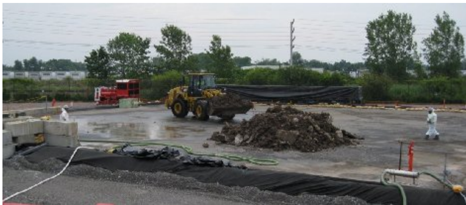
Figure 5: Linde FUSRAP Site loading area.
