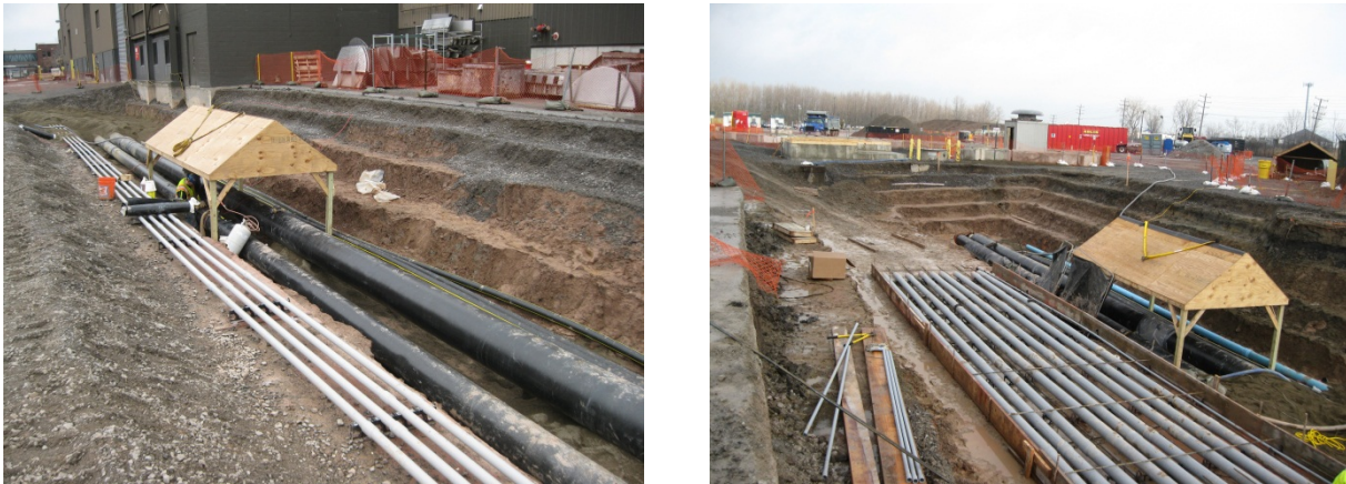
Fig. 7. Performing direct buried utility installation.
