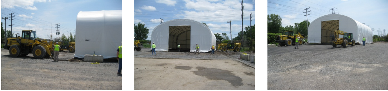
Fig. 3. From left to right, phase one, phase two, and phase three of the salt barn move.
