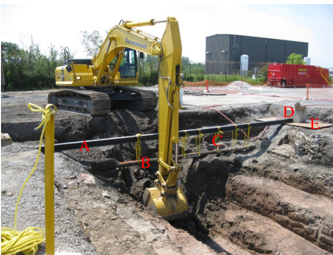
Fig. 5. Structural support of an active ductile iron water line.
