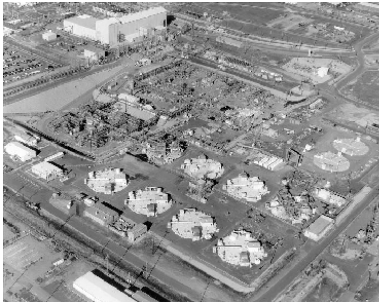
Fig. 3 Typical storage tanks at Savannah River Site
