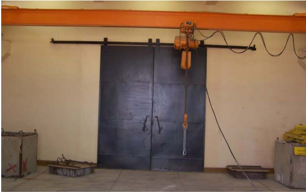
Figure 2: WORKING AREA STORAGE FACILITY AFTER EMPTYING ITS CONTENTS
