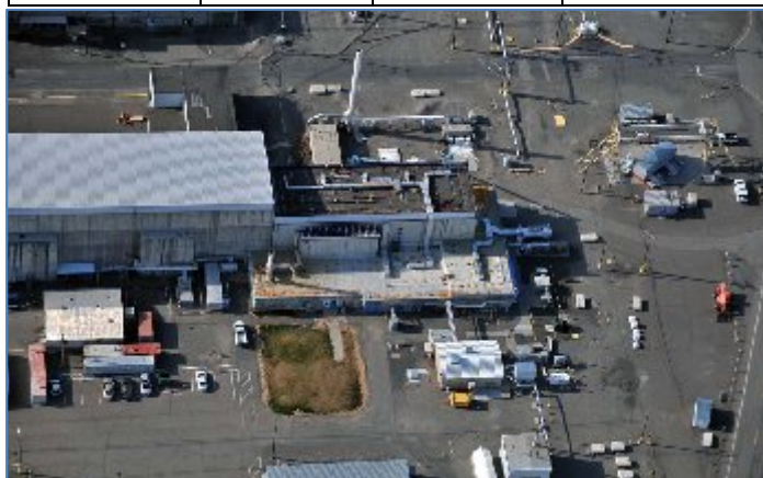
Fig. 1. Waste Encapsulation Storage Facility
