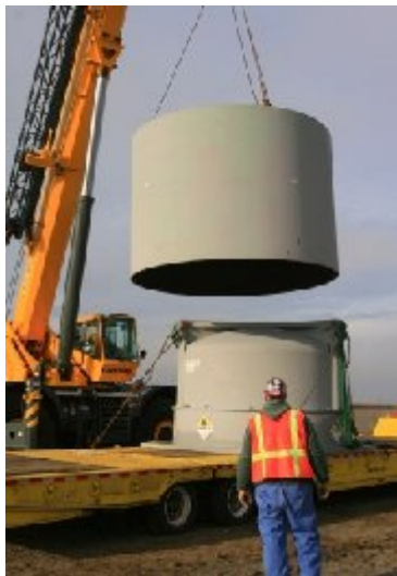
Fig. 4. Reactor Compartments being offloaded at the LLBG.
