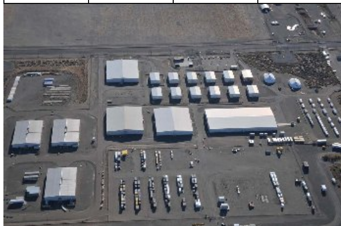
Fig. 3. Central Waste Complex/Low-Level Burial
