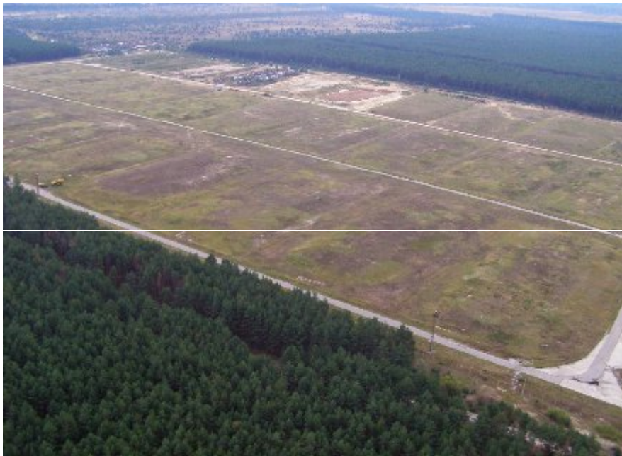
Fig. 2: Aerial view of RWDF Buryakovka
