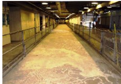
Photo 6 – Basin Segment After Grouting
