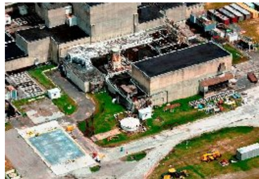
Photo 4 – Building 710-C After
