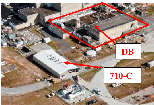
Photo 3 – Building 710-C Before
