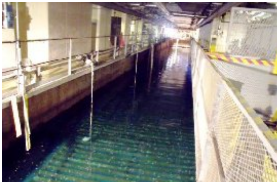
Photo 5 – Basin Segment Before Grouting
