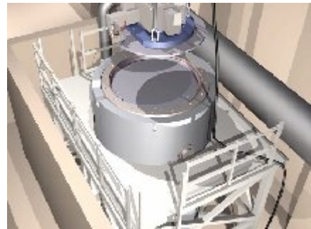
Figure 10, Placing Lid on RWC
