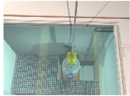
Figure 8, Transfer Cask in Pool
