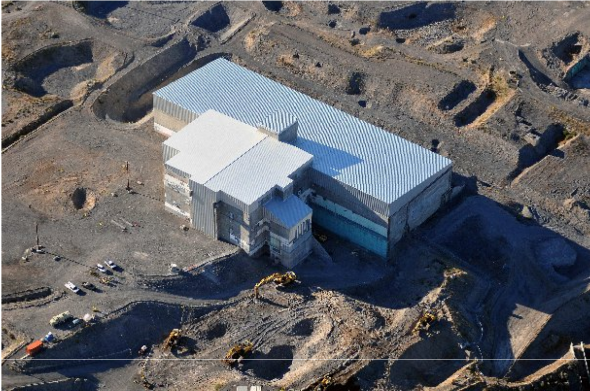
Fig. 7. 105-N and 109-N Building SSEs with simplified shed roof designs (2012).
