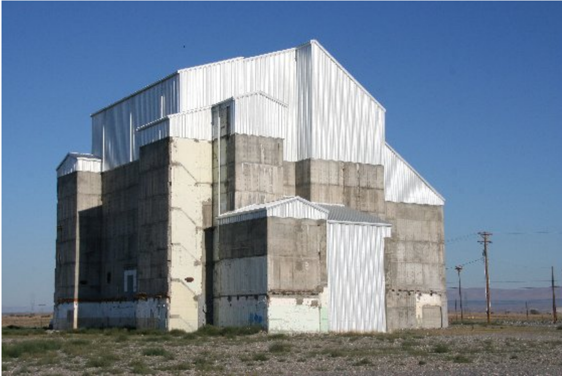
Fig. 3. 105-DR and 105-F (above) Reactor SSEs were built to the same peaked-roof design.
