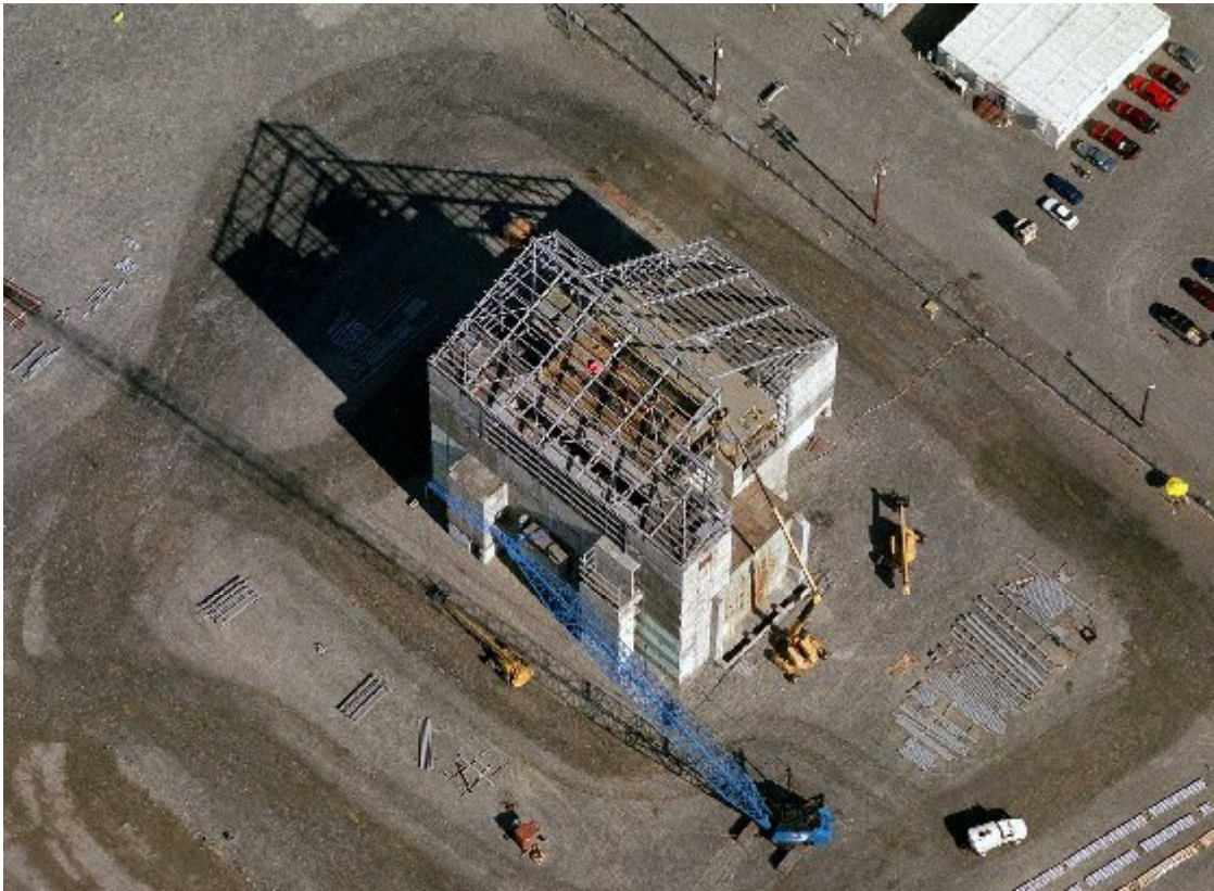
Fig. 5. H Reactor SSE showing streamlined roofline design with structural steel erected.
